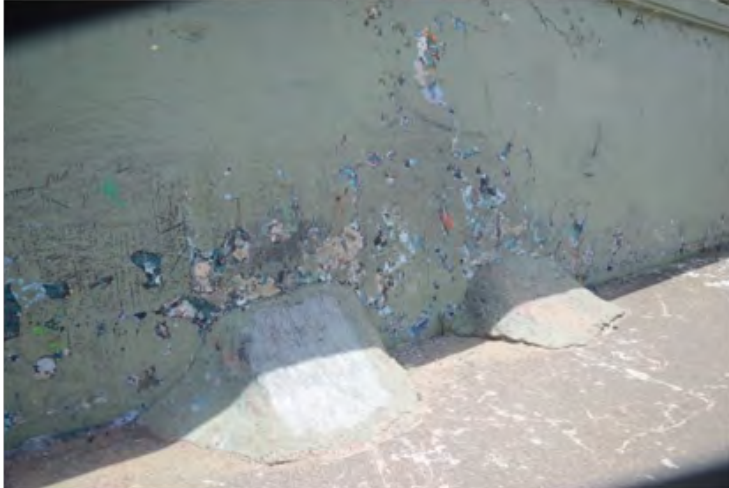
Figure 16. User added concrete ramps at Newcastle Beach skatepark.
